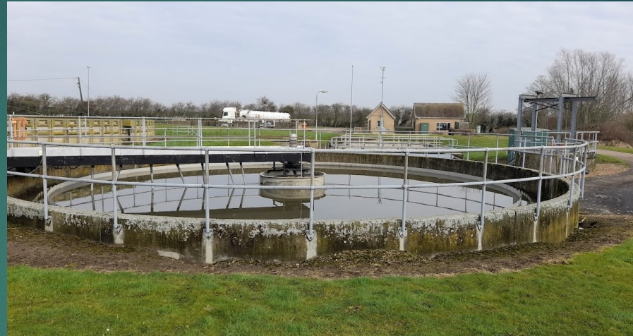
Storm tank overflow 3 March 2022
